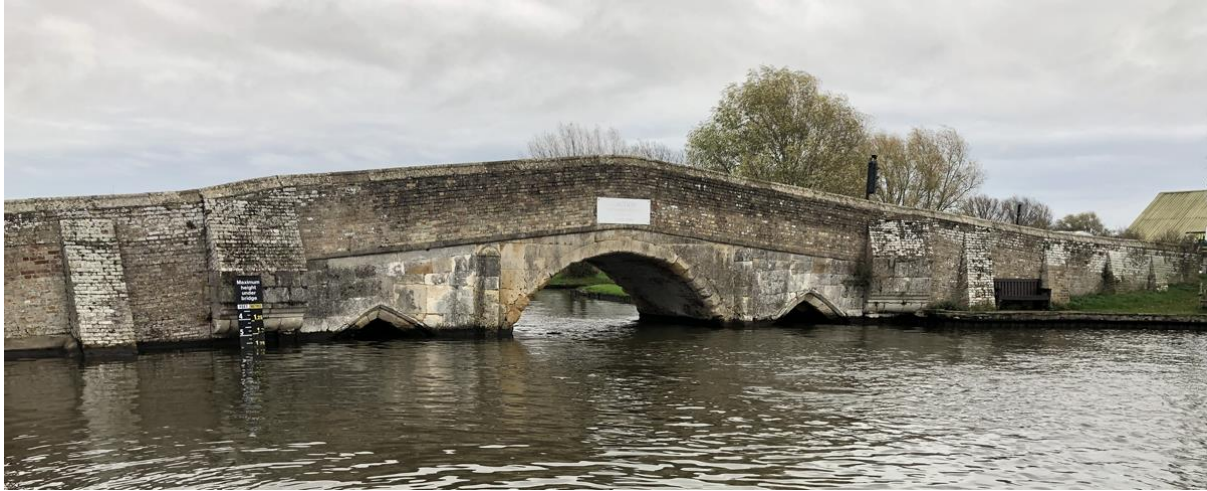
Potter Heigham Bridge
