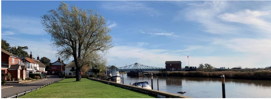
Reedham swing railway bridge over the River Yare
