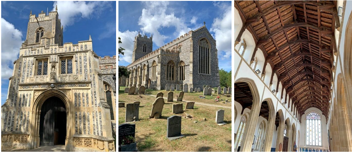
South porch, View from the south-east and Hammerbeam roof to the nave
