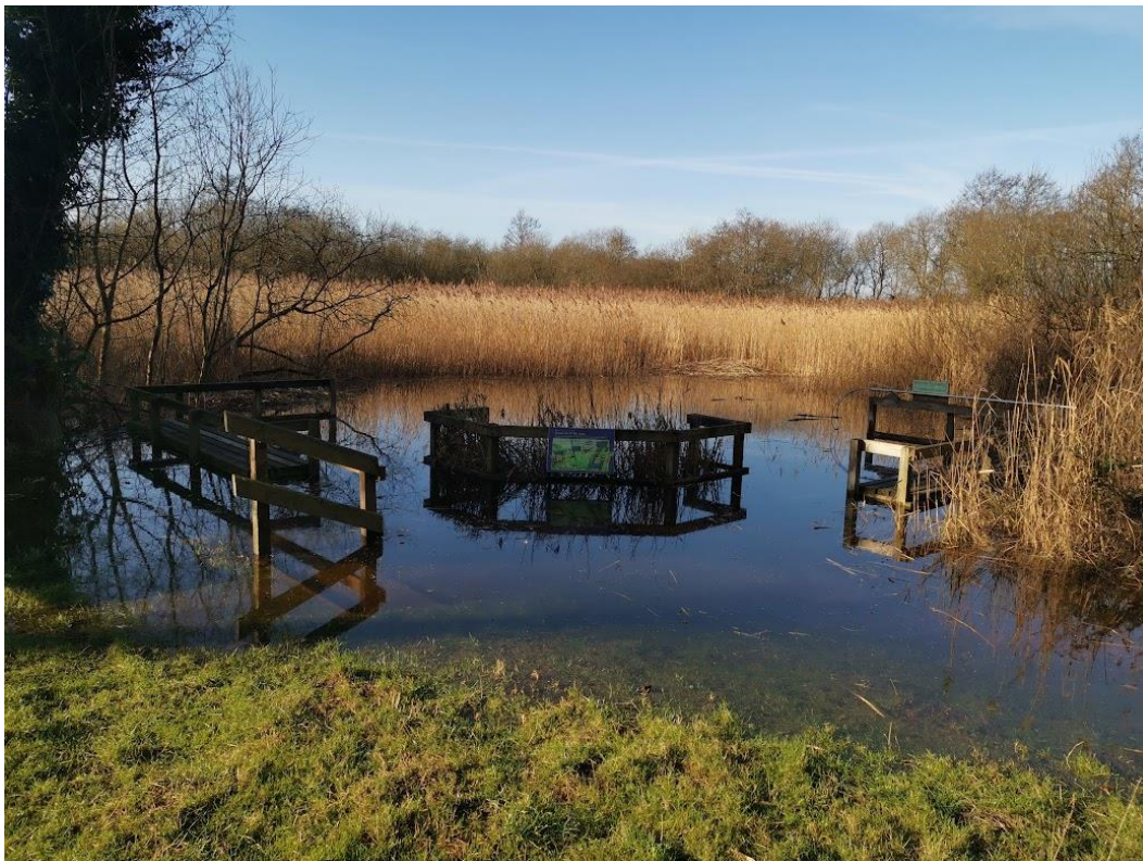
A flooded pond dipping platform at Strumpshaw Fen in January
