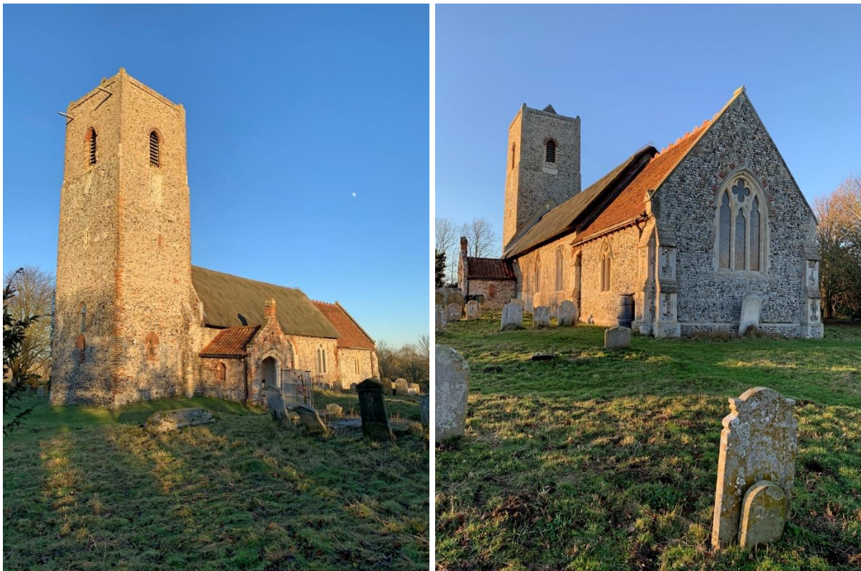
View from the south-west with the 16 th century tower and view from the south-east.
