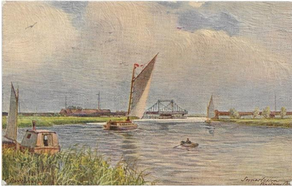
Somerleyton Railway Bridge
