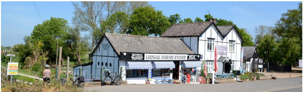
Existing buildings adjacent to Ludham Bridge
