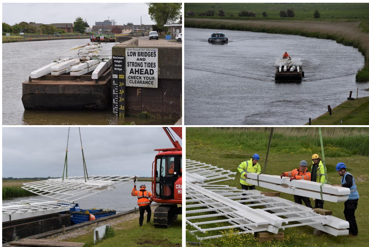
Stocks and sails being transported along the River Bure and unloaded at the mill
