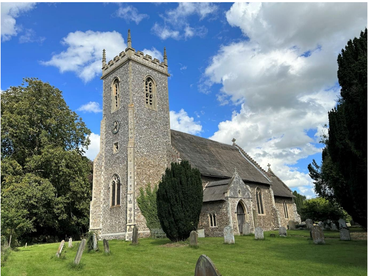
View of the church from the south-west
