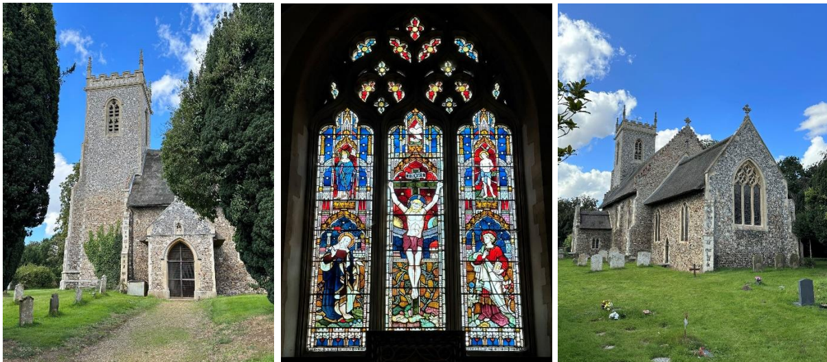
West tower and south porch; Stained glass to east window; View from south-east
