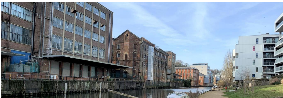
Existing vacant buildings at the Carrow Works site along the River Wensum, Norwich
