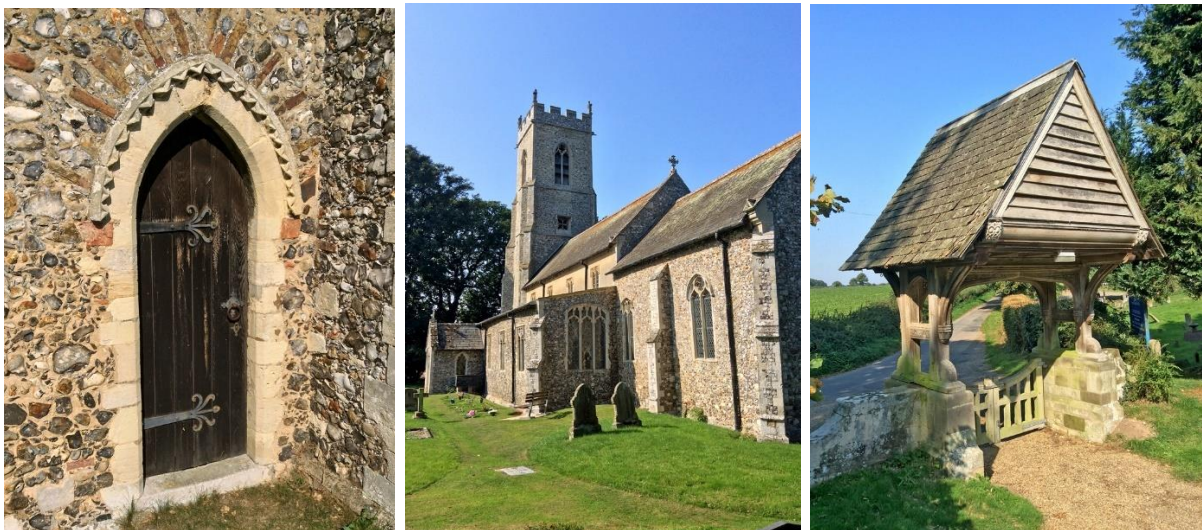
13 th century priest's door with dog-tooth arch; West tower; Lychgate to churchyard.
