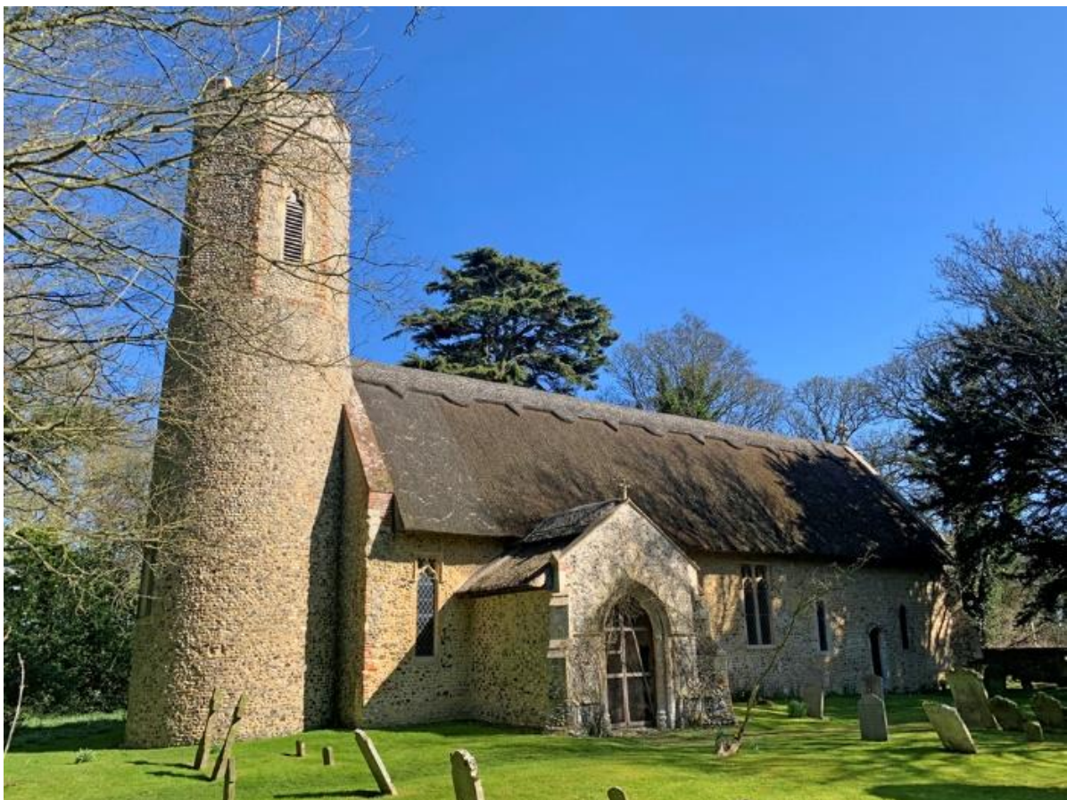
View of the church from the south-west
