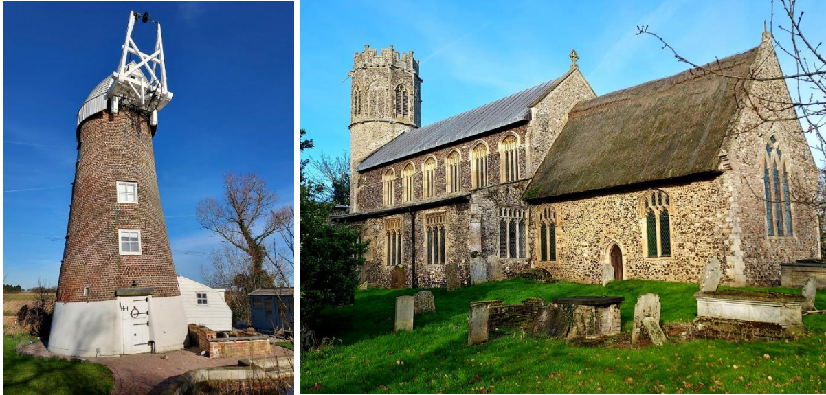
High Drainage Mill and Church of St Nicholas, Potter Heigham
