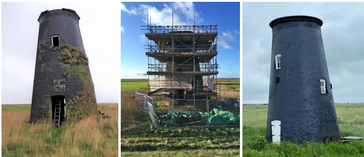
Six Mile House before, during and after restoration
