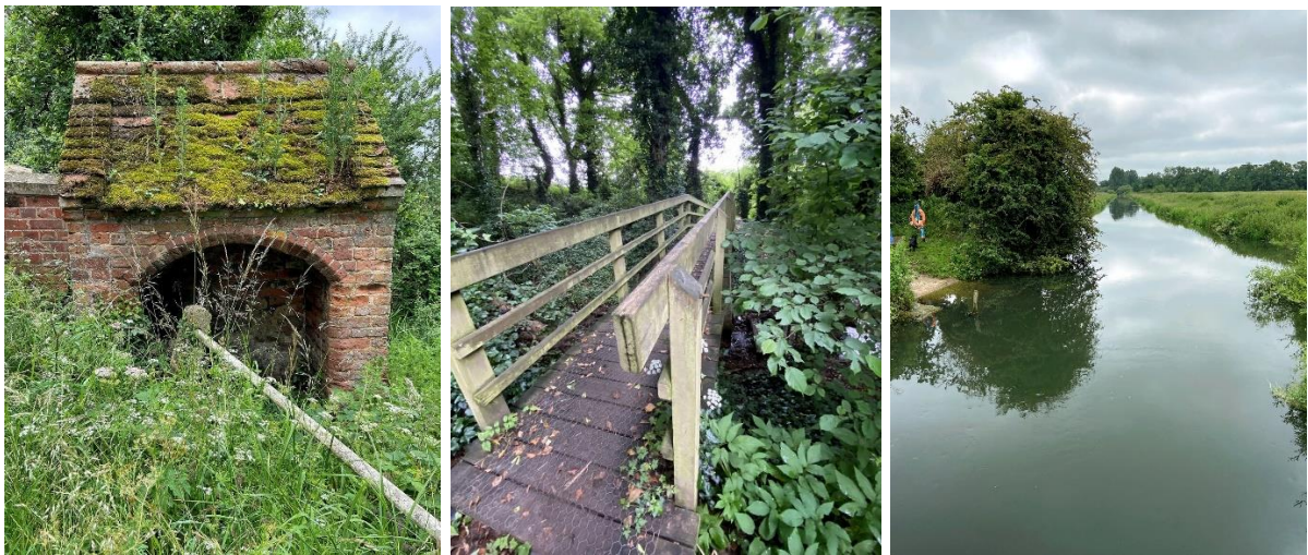
Toll collectors' shelter at Mayton Bridge; wooden footbridge and the River Bure
