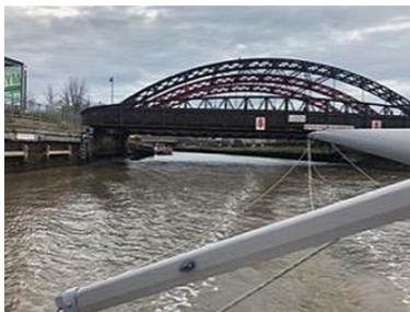
Vauxhall Bridge at Yarmouth has a clearance of 6.09 feet at High Water Springs with a height range between Springs and Neaps of about 2.4 feet. So, with St Helen needing 6.2 feet minimum, a passage on most days at High Water would be alright. I would take into consideration whether the wind on the North Sea had been strong from the North or Northeast for a few days as
