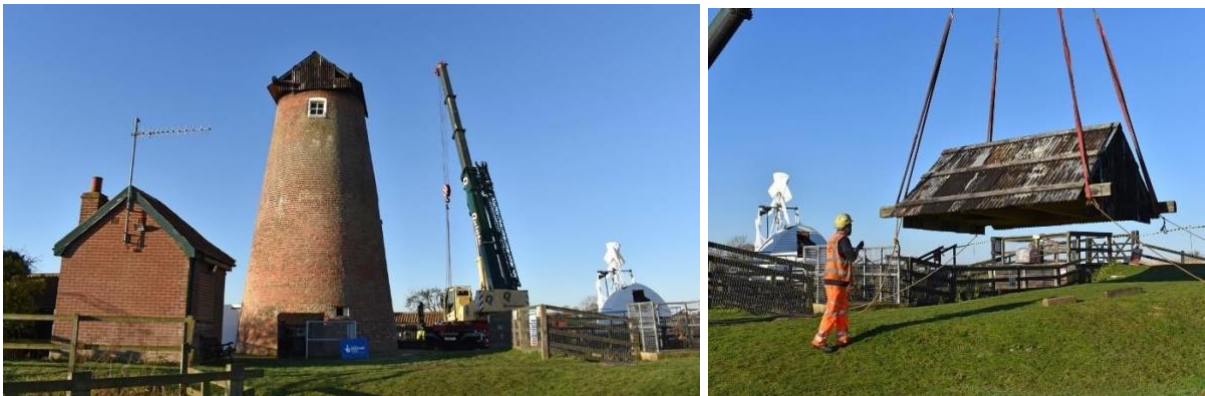
Stracey Arms Mill with its temporary roof being removed prior to fitting of the new cap
