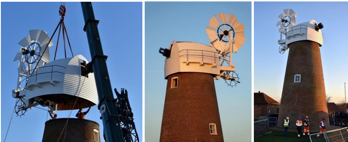
The new cap being hoisted into place by crane and after fitting in position. All images © Norfolk Windmills Trust
